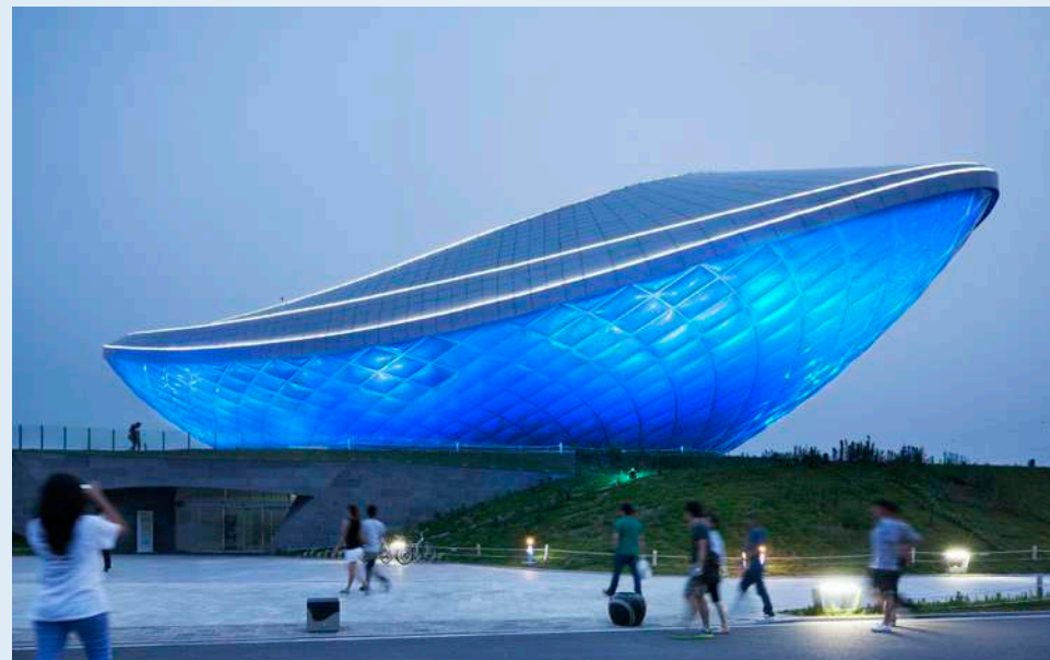
ARC River Cultural Pavilion, Daegu, South Korea
